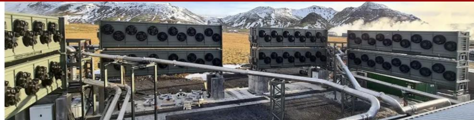
"Orca," Climeworks' new facility in Iceland, can capture 4,000 tons of carbon dioxide per year. Business Wire via AP
